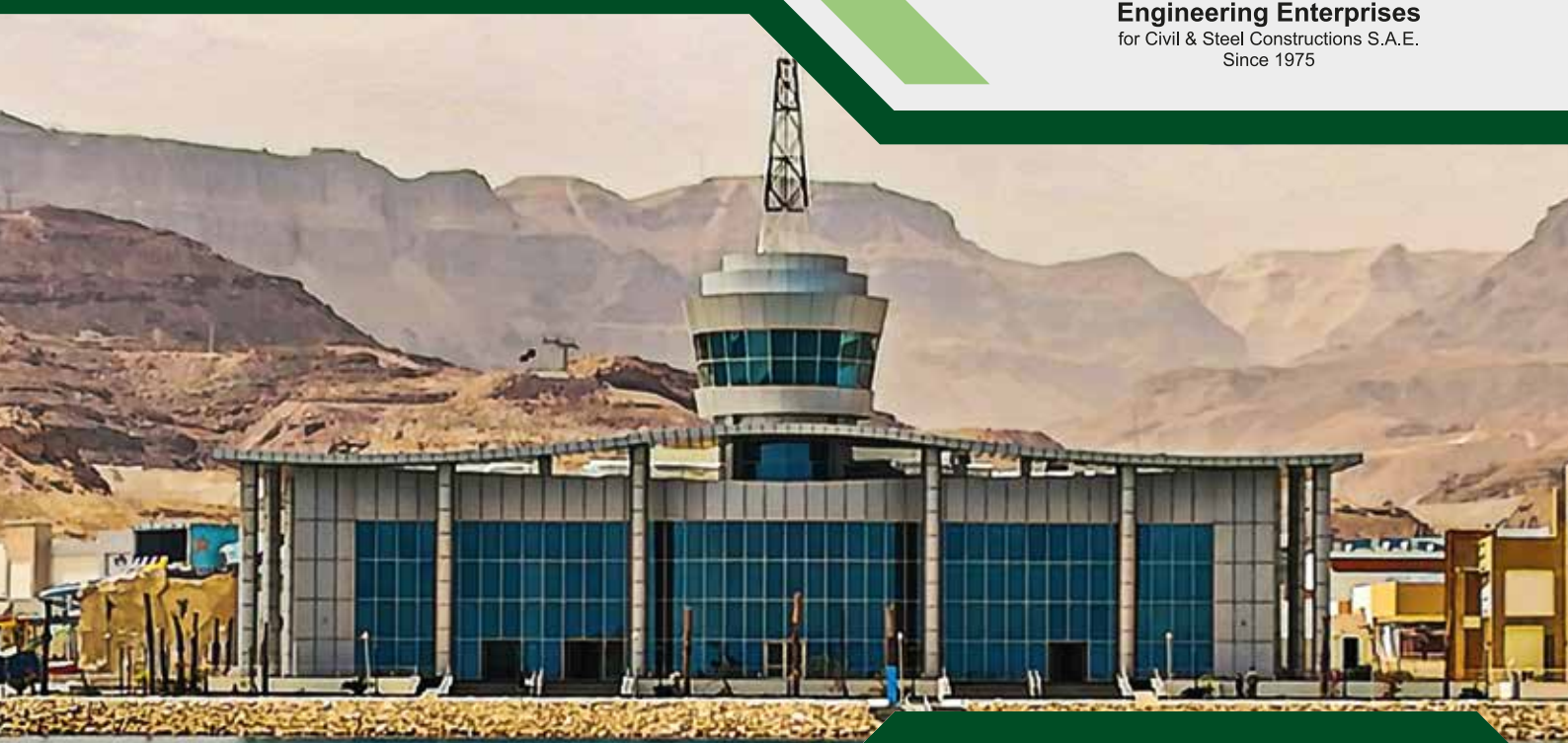
SEAPORT BUILDING - AIN EL SOKHNA
